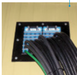
Wall penetration in process building: Roxtec G frame solution for cables and pipe entries through walls.
