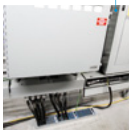
Floor penetrations: Roxtec G frames are welded or bolted to floors as a space-saving solution for large quantities of cables and/or pipes.
